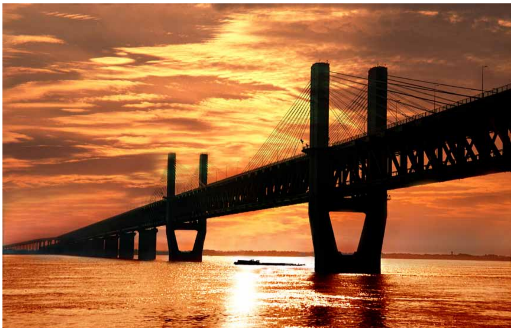
The Wuhu Yangtze River Bridge is a transport pivot linking the south and north of Anhui.
